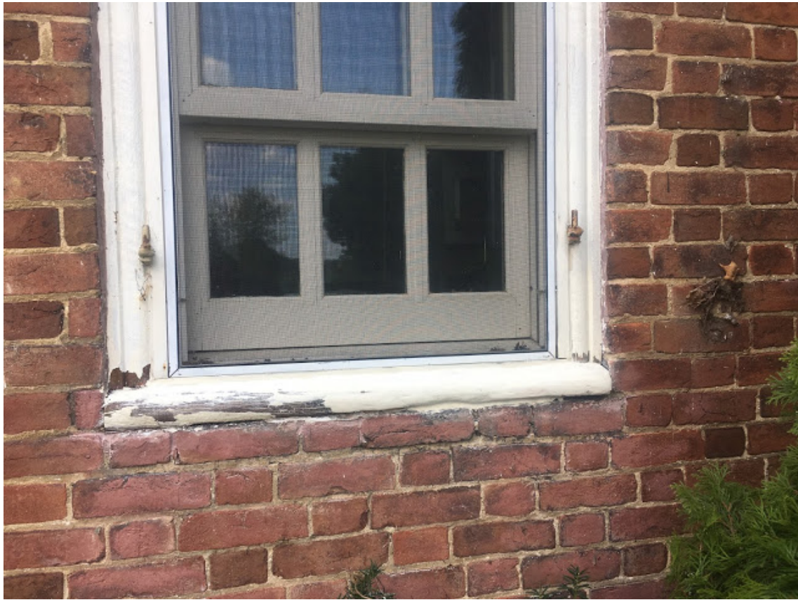
This is how the sill looked after it was dried and sanded.
